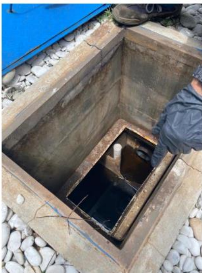
Gambar 7. Unit Filter Anaerob Biopal
