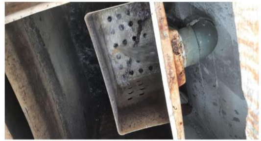
Gambar 5. Bar Screen Biopal
