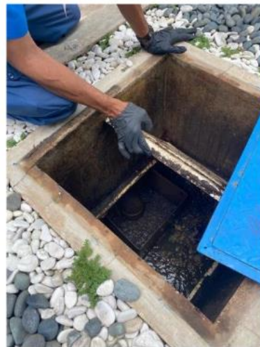
Gambar 6. Unit Sedimentasi 1 Biopal
