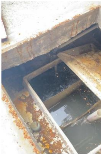
Gambar 8. Unit Filter Aerob Biopal
